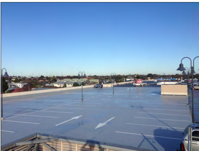
Finished Car Park
