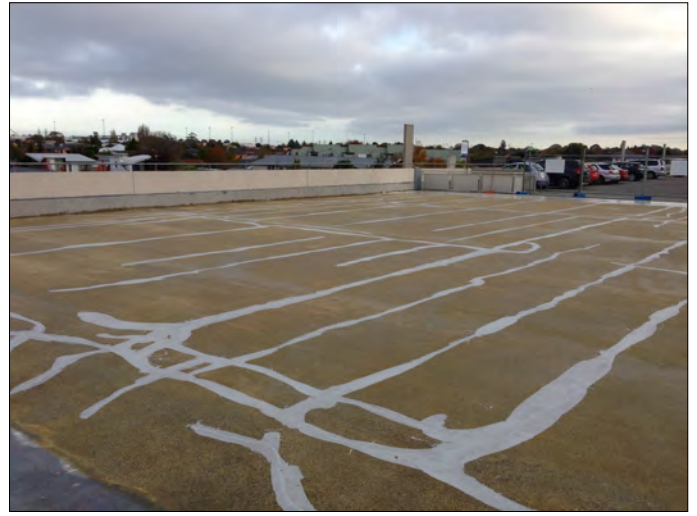
Crack Repair
