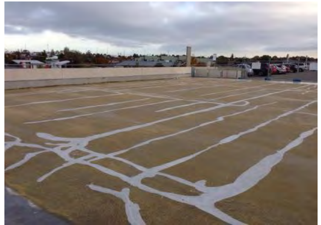
Crack repair
